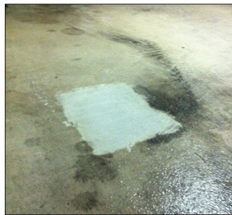
Carpark Epoxy Floor
